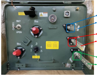
(a) Split-phase distribution transformer
